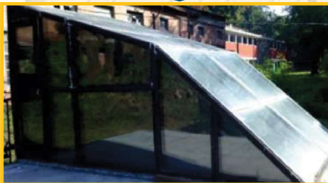
Head based storage Solar Kiln
